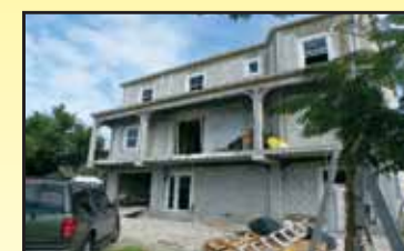
BRAND NEW 4/4 HOME BEING BUILT in Tavernier. Why buy existing finishes when you can choose your own? Large home on great canal with good access to the gulf; near Snake Creek ocean access.
