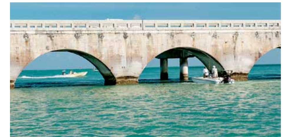
Following the fish through the concrete arch of the former Florida East Coast Railway Extension.
