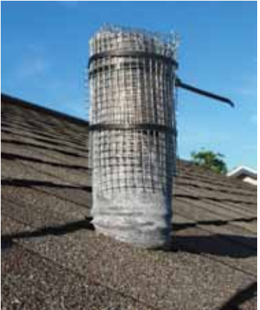
Cover roof vent pipes with hardware cloth and wire mesh to prevent entry into buildings by Cuban Tree Frogs. Credit: UF/IFAS
